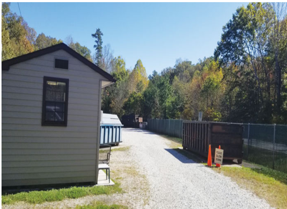
A typical rural citizen's convenience center. One-way traffic flow and location partially in DOT right-of-way makes efficient use of real estate. Images courtesy of SCS Engineers.
