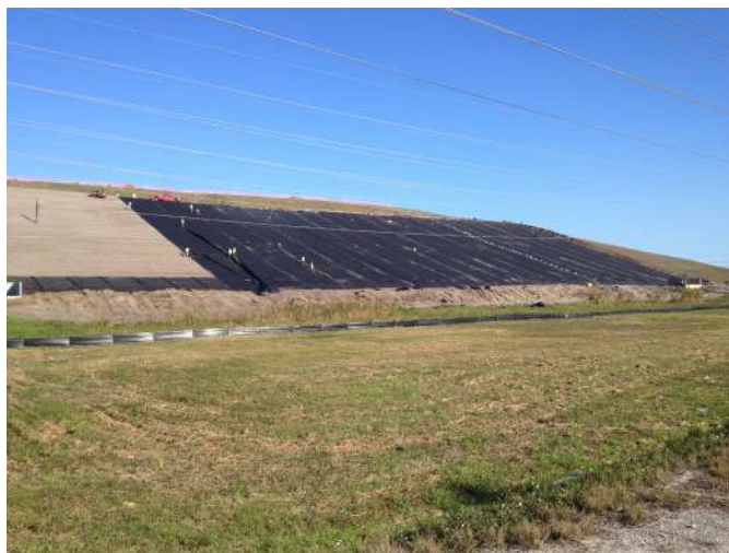
Figure 2 - Final cover geomembrane installation in progress.
