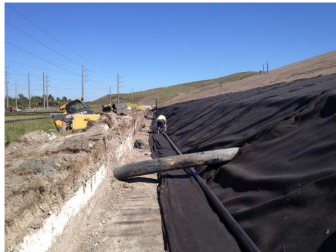
Figure 1 - LTDS under construction at the toe of the landfill slope.
