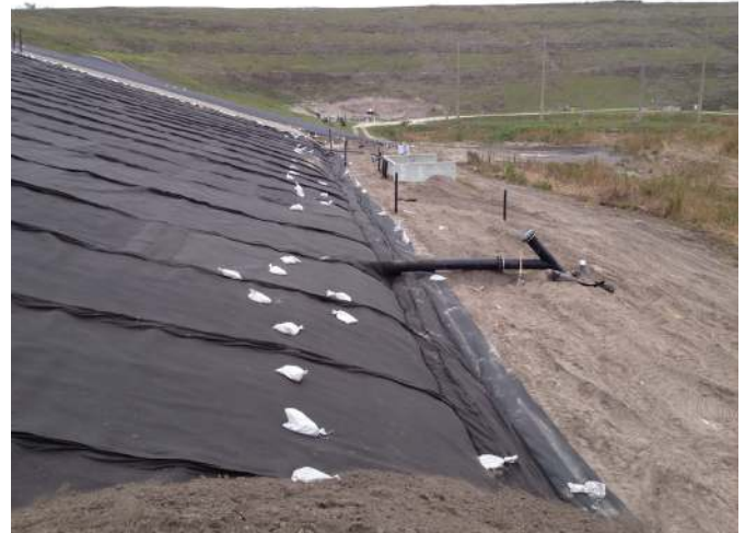
Figure 3 - RTDS completed near the toe of the landfill slope.
