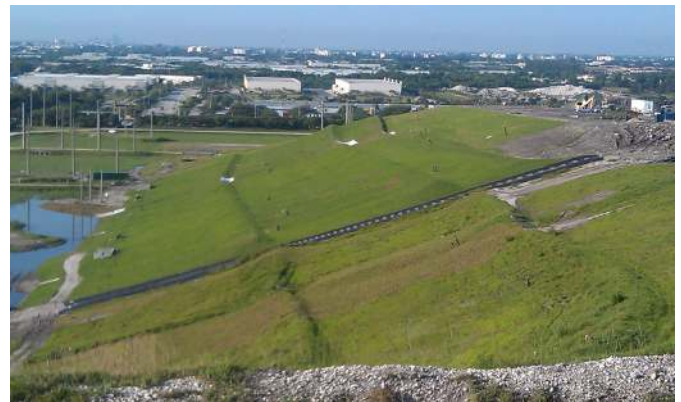
Figure 4 - Final condition with drainage swales and downchutes.
