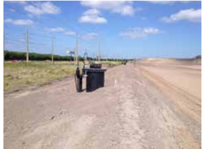
Figure 2 Gas condensate sump at completion of perimeter berm.
