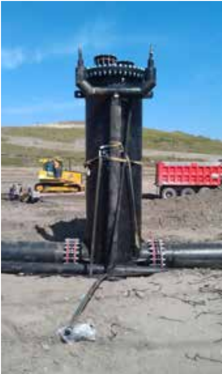
Figure 1 Construction of gas header, gas condensate sump, condensate force main, and compressed air lines in landfill perimeter berm.
