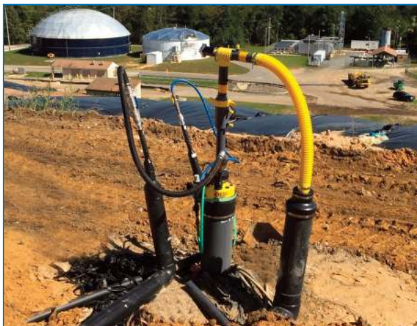
Figure 2. Landfill gas extraction well and pump for liquids removal.
