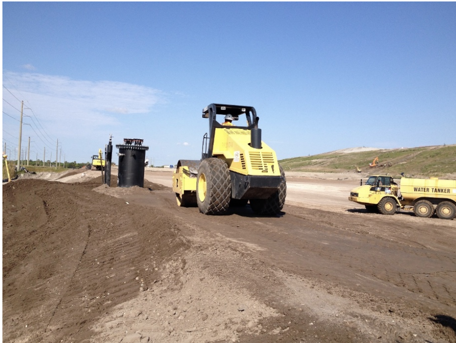
Construction of perimeter berm in vicinity of condensate sump.
