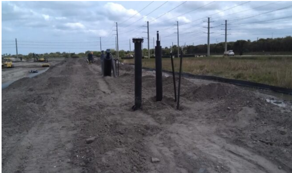
Stubouts for lateral header, condensate force main, and compressed air lines for future extension on landfill slope.
