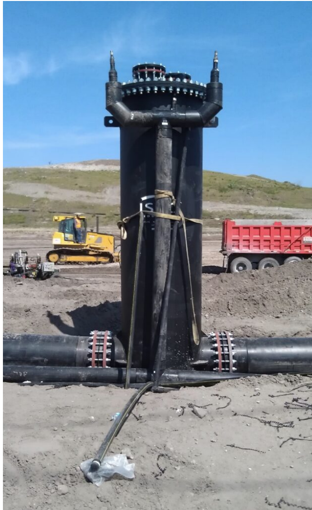
Condensate sump with gas header connections in perimeter berm (lower portion of the sump not shown in the photo).
