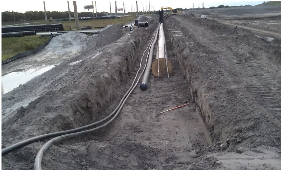
Gas header, Condensate force main, and compressed air lines in perimeter berm.
