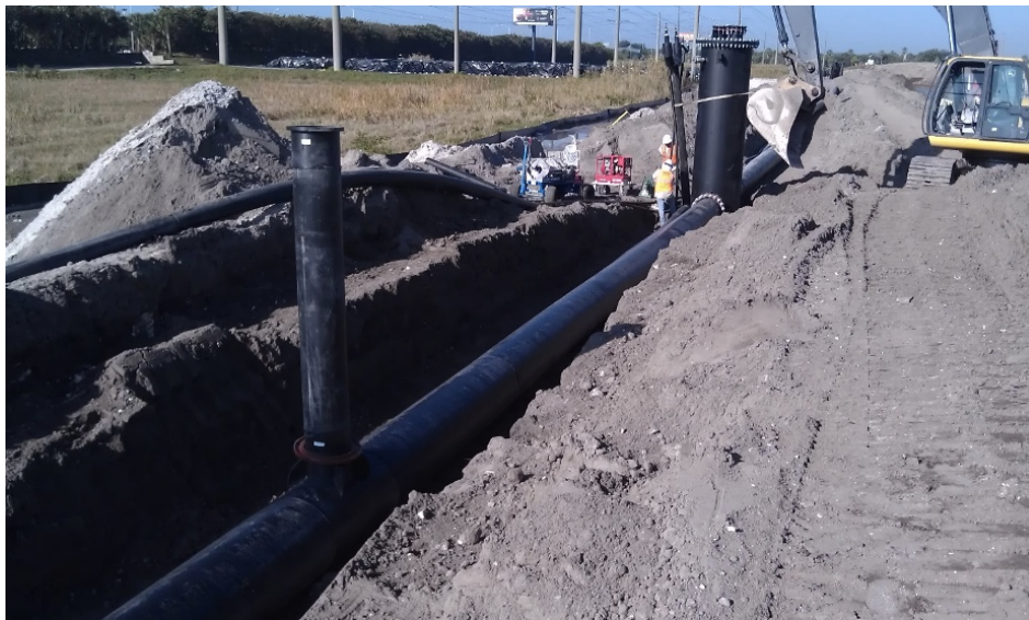
Stubout for a lateral header on the gas header in perimeter berm.
