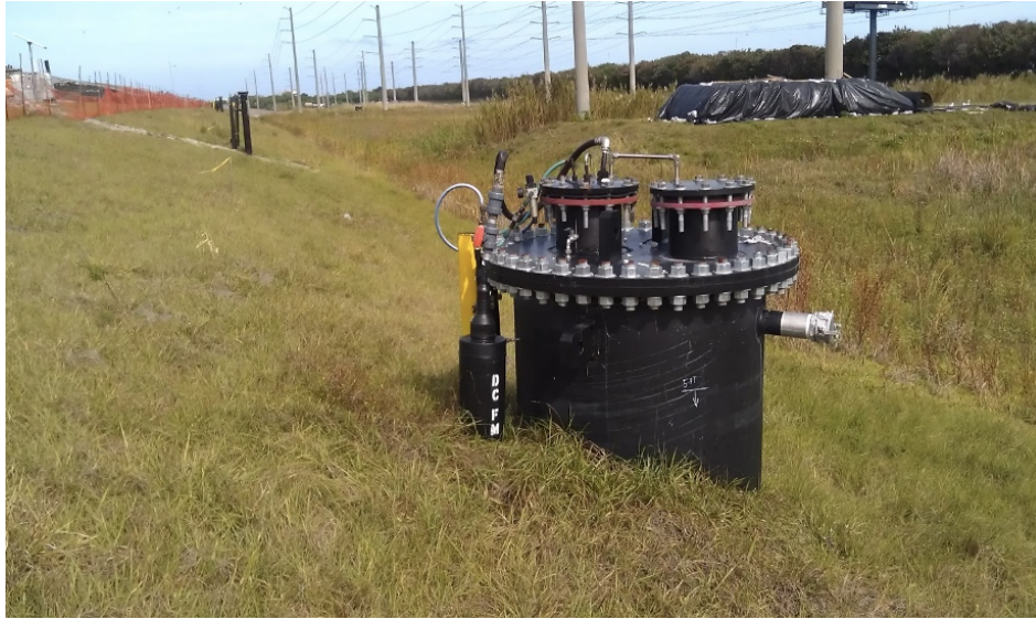
Condensate sump in perimeter berm.
