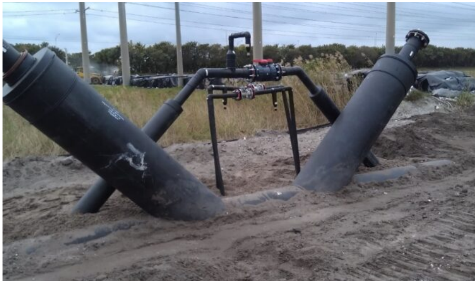
Gas header cleanouts, exposed condensate force main with isolation valve and air release valve, exposed compressed air lines with isolation valves and liquid removal valves.
