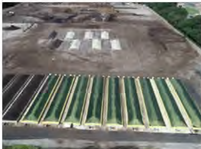
Aerated static piles are used at a compost site utilized by Maryland's Prince George's County.
