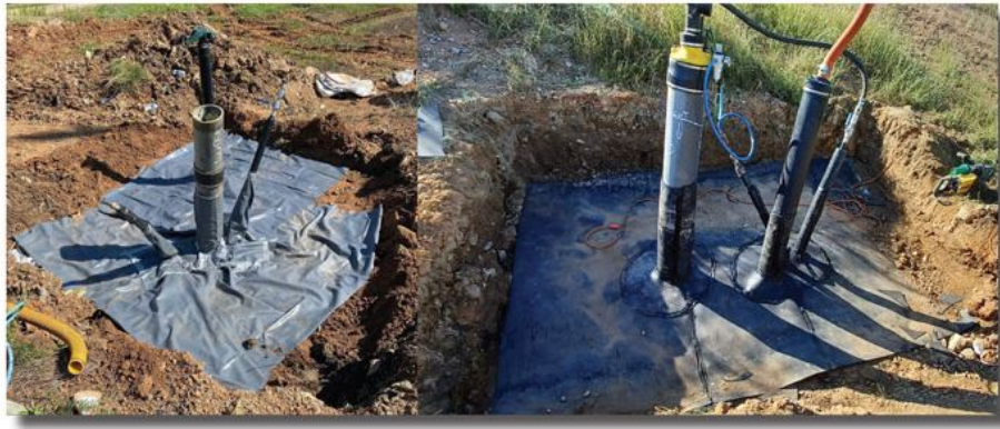
Above and right: Penetration corrective action using prefabricated seal.
