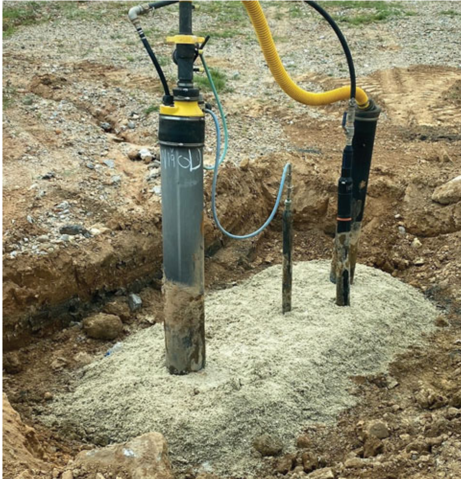
Penetration corrective action using bentonite.
