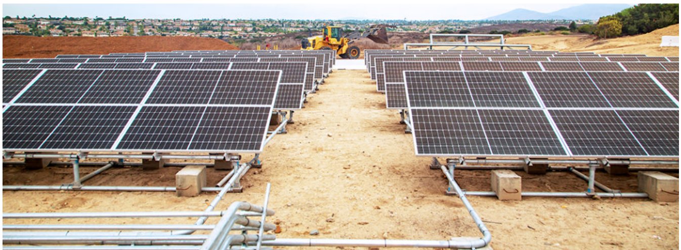
There are 168 solar panels arranged in 14 solar arrays that generate 43 kW of electricity, and 573 kW of battery storage.
