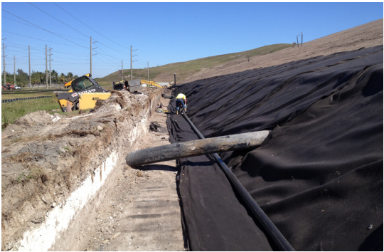
Photo 2: LTDS under construction below cover geomembrane
