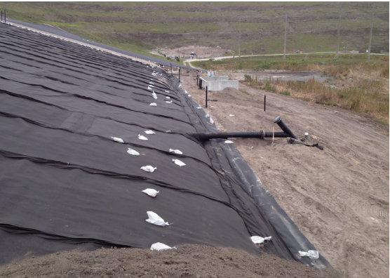
Photo4: RTDS completed above Cover Geocomposite
