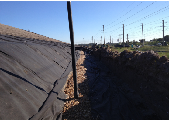
Photo 3: Vacuum pipe connected to LTDS pipe.
