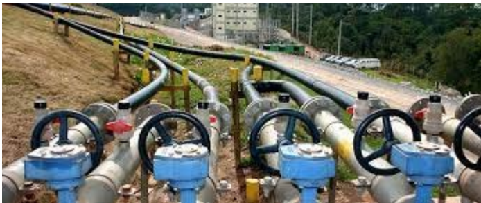
LFG collection system
