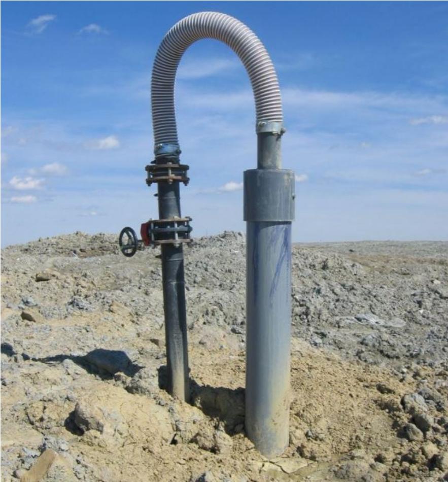
One of about 300 landfill gas wellheads at the Rumpke Sanitary Landfill, which recover the landfill gas.
