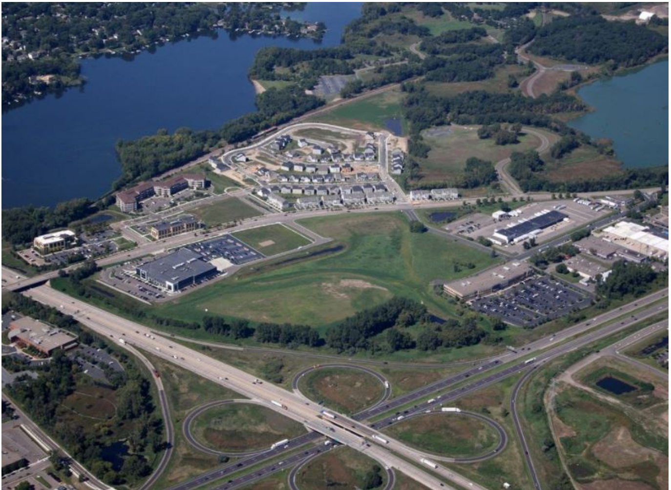
The New Brighton Exchange project in New Brighton, MN. Barr Engineering worked with the city to clean up and develop the area, which had included two former dumps, two Superfund sites, and several petroleum-release sites. Most of the area is now redeveloped and includes office buildings, apartments, and parks.
