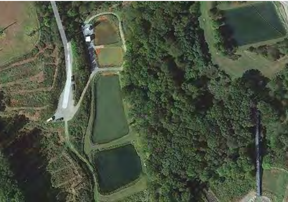
Water treatment ponds show improvement. (Photo: SCS Engineers)
