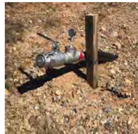
Figure 2 - Pressure gauges and cleanouts are beneficial for troubleshooting dewatering forcemain systems.
