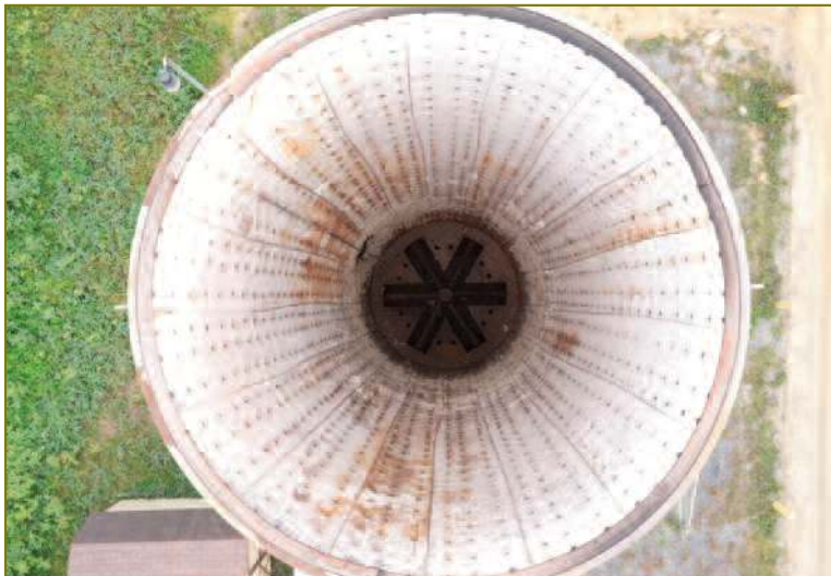
Figure 3. Drone Inspection of a Flare Stack.
