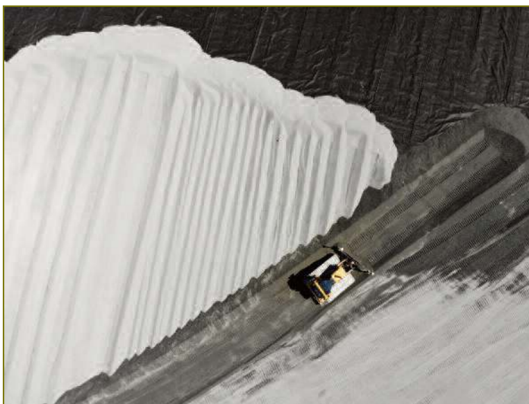
Figure 4. Drone Used in Construction Quality Assurance (CQA) Services.
